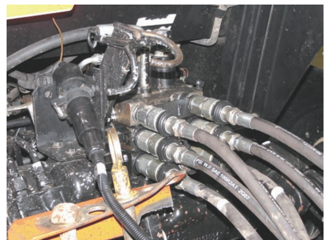
Disconnect Hydraulic Hoses
