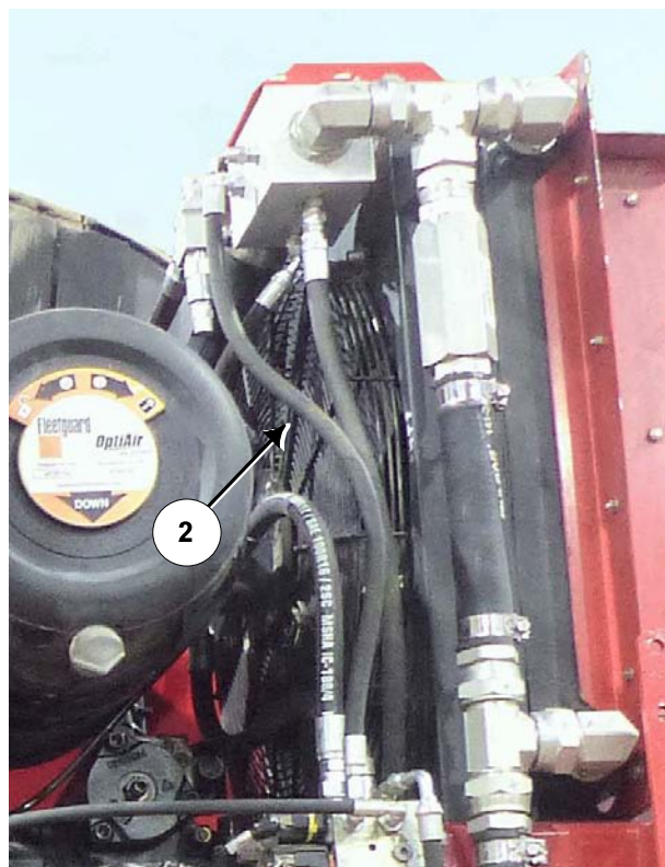
Clear Debris from Oil Cooler Fan
