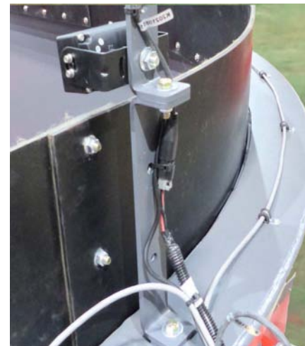
Attach Cables to Top of Tank Rim
