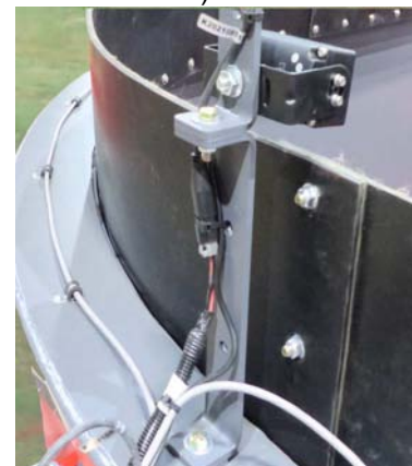
Attach Cables to Top of Tank Rim
