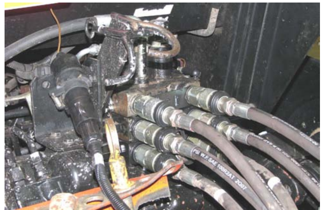
Disconnect Hydraulic Hoses & Electrical
