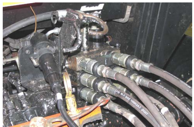
Attach Hydraulics and Electrical
