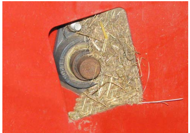
Remove Material - Lower Chain Bearing
