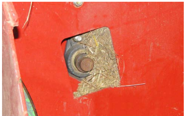
Remove Material - Lower Chain Bearing
