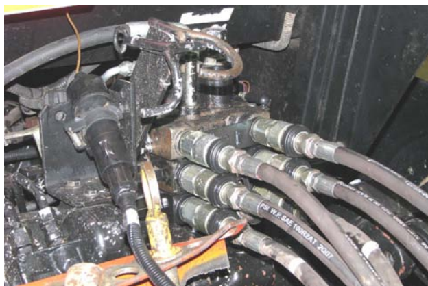
Attach Hydraulics and Electrical
