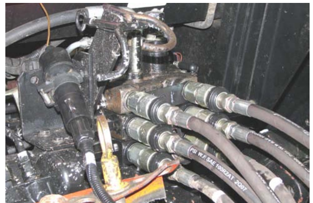
Attach Hydraulics and Electrical
