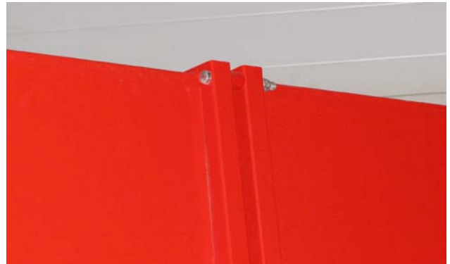
Remove Fastener and Spacer Between Walls 215104
