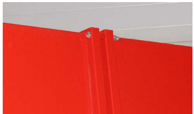
Remove Fastener and Spacer Between Walls
