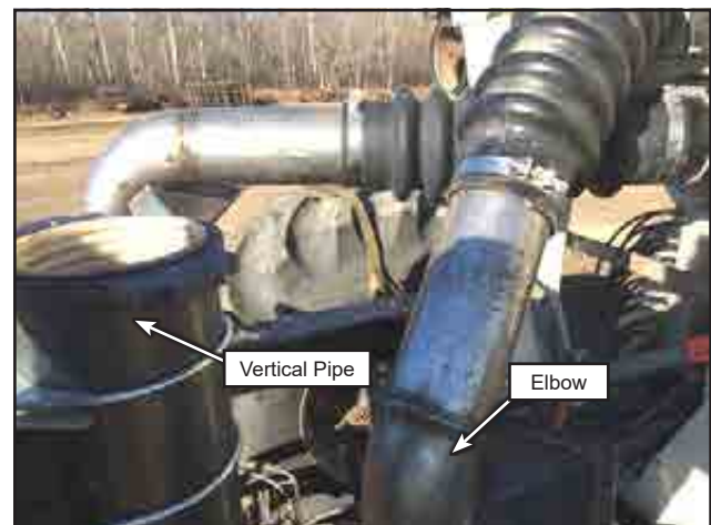
Figure 1.14 - Elbow Removed from Vertical Pipe
