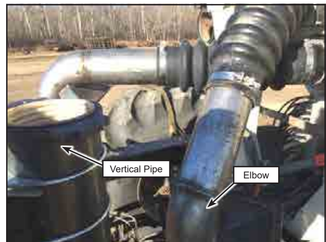
Figure 1.13 - Elbow Removed from Vertical Pipe
